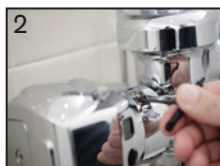
2 Secure the mounting clamp (two screws)
